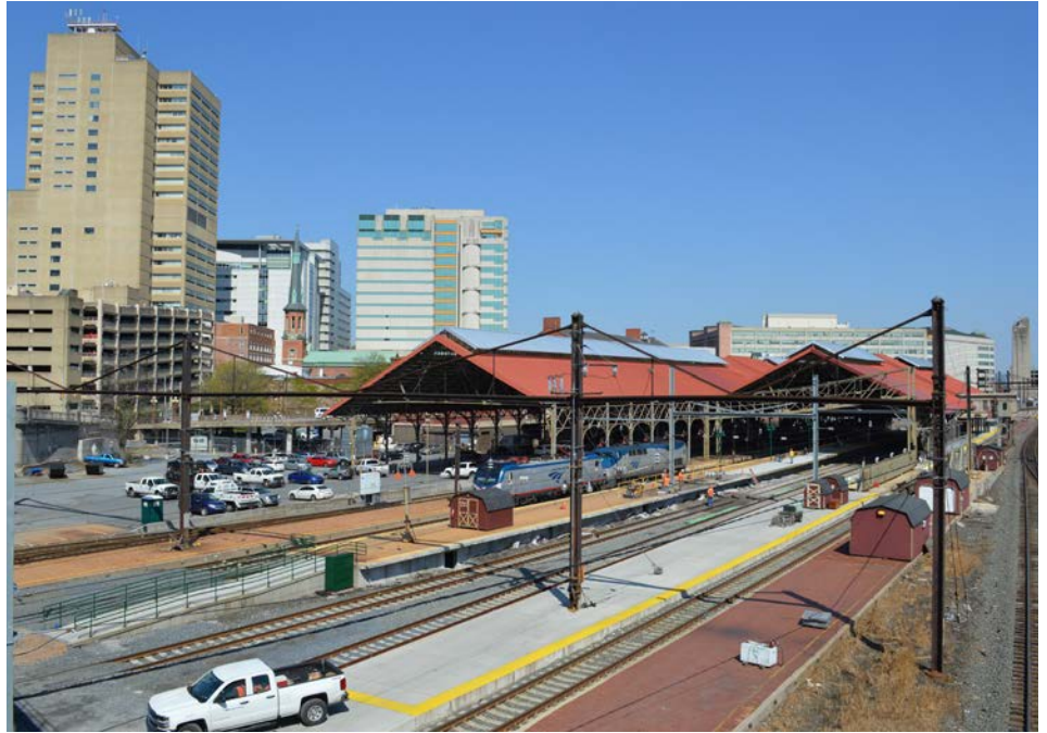
The catenary support structures, seen in the foreground of this photograph, were constructed by the Pennsylvania Railroad during the 1930s electrification program.
