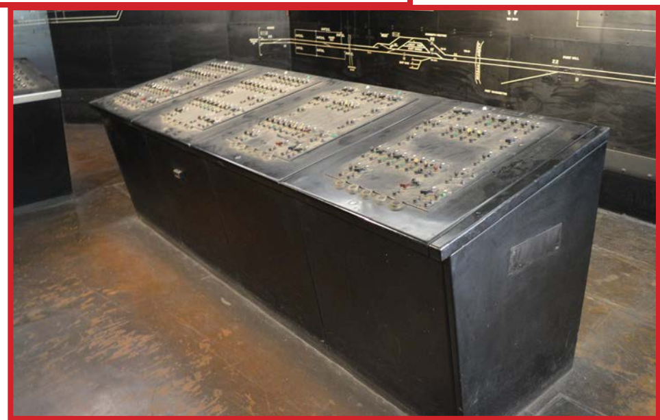
The supervisory control units manufactured by Westinghouse feature a control panel for each power substation along the lines. The control units were specially configured to direct the function of various "apparatus" within each power station - including circuit breakers to turn power on or off, and transformers to convert high power to the appropriate voltage for operating the train equipment.
