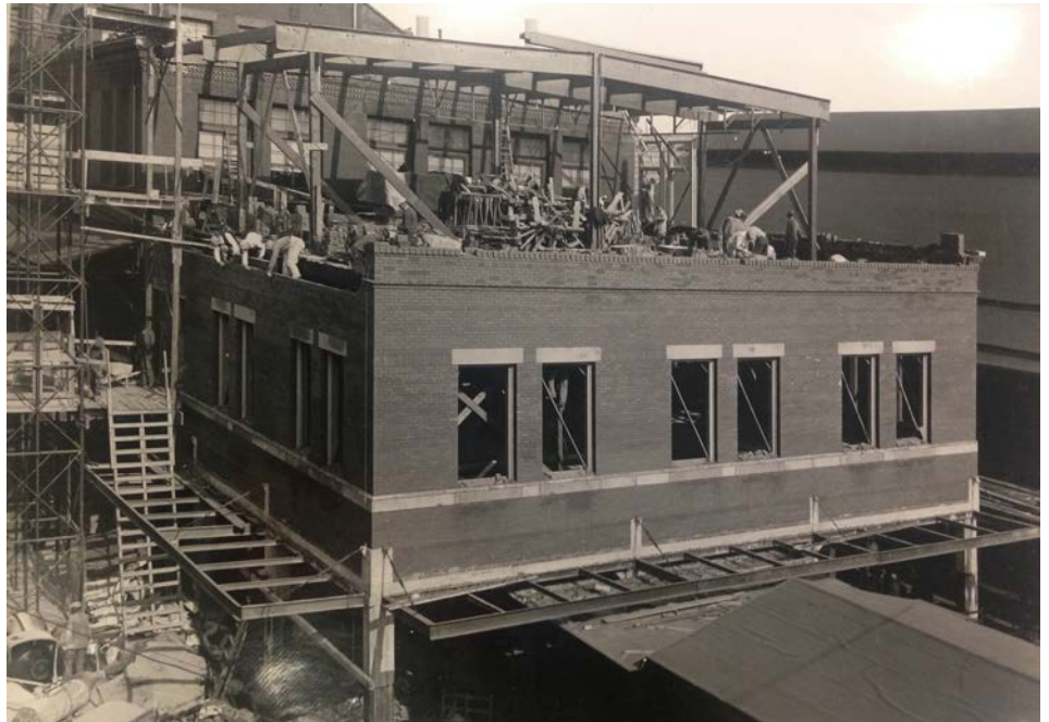
This addition, as seen under construction in 1936, was designed to hold interlocking equipment on the main floor, and the Power Director's Room on the second floor.
