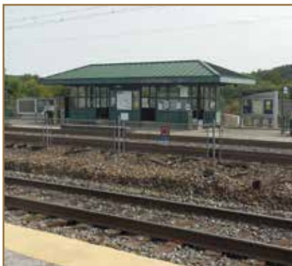
▼ View of the Downingtown Station eastbound passenger shelter in 2020.
