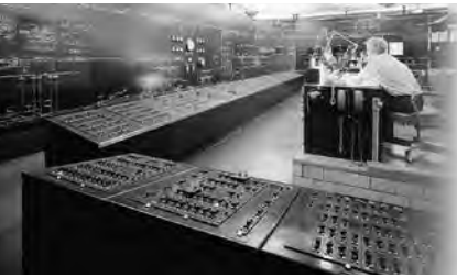
image courtesy of HAER
